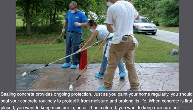
particularly concrete which will be subject to freezing and thawing. The major way to make concrete more resistant to freeze/thaw cycles is through air entrainment — the purposeful addition of tiny air bubbles into the concrete during batching. After the concrete
