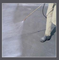
The goal is to keep concrete cool and moist so it gains strength slowly, but efficiently. Laboratory tests show that moist-cured concrete can be twice as strong as concrete cured in a dry environment.
