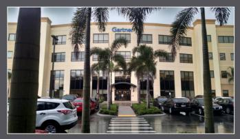
Tilt-up is the advanced construction method for low to mid-rise structures. Load-bearing concrete wall panels are cast horizontally on site and then tilted up into position.
